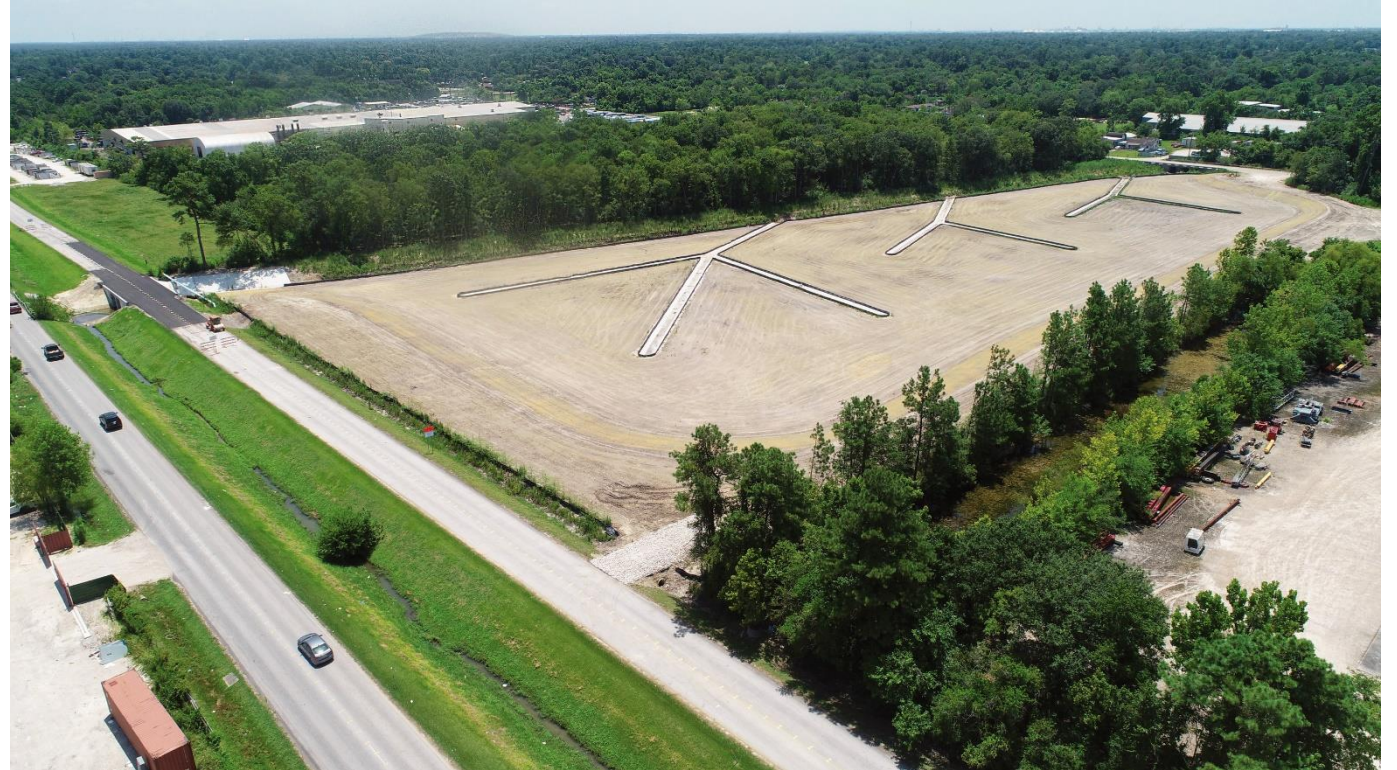
Picture: Completed Little York Stormwater Detention Basin
